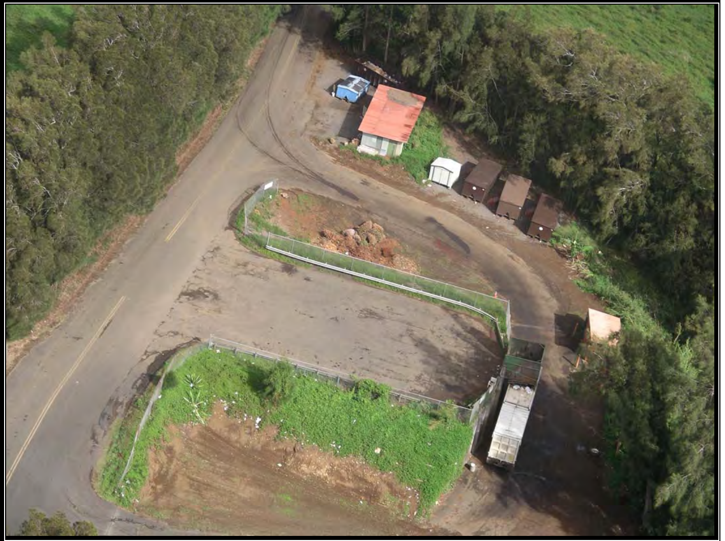
Figure 1b North Kohala Existing Convenience Center Location Airphoto
