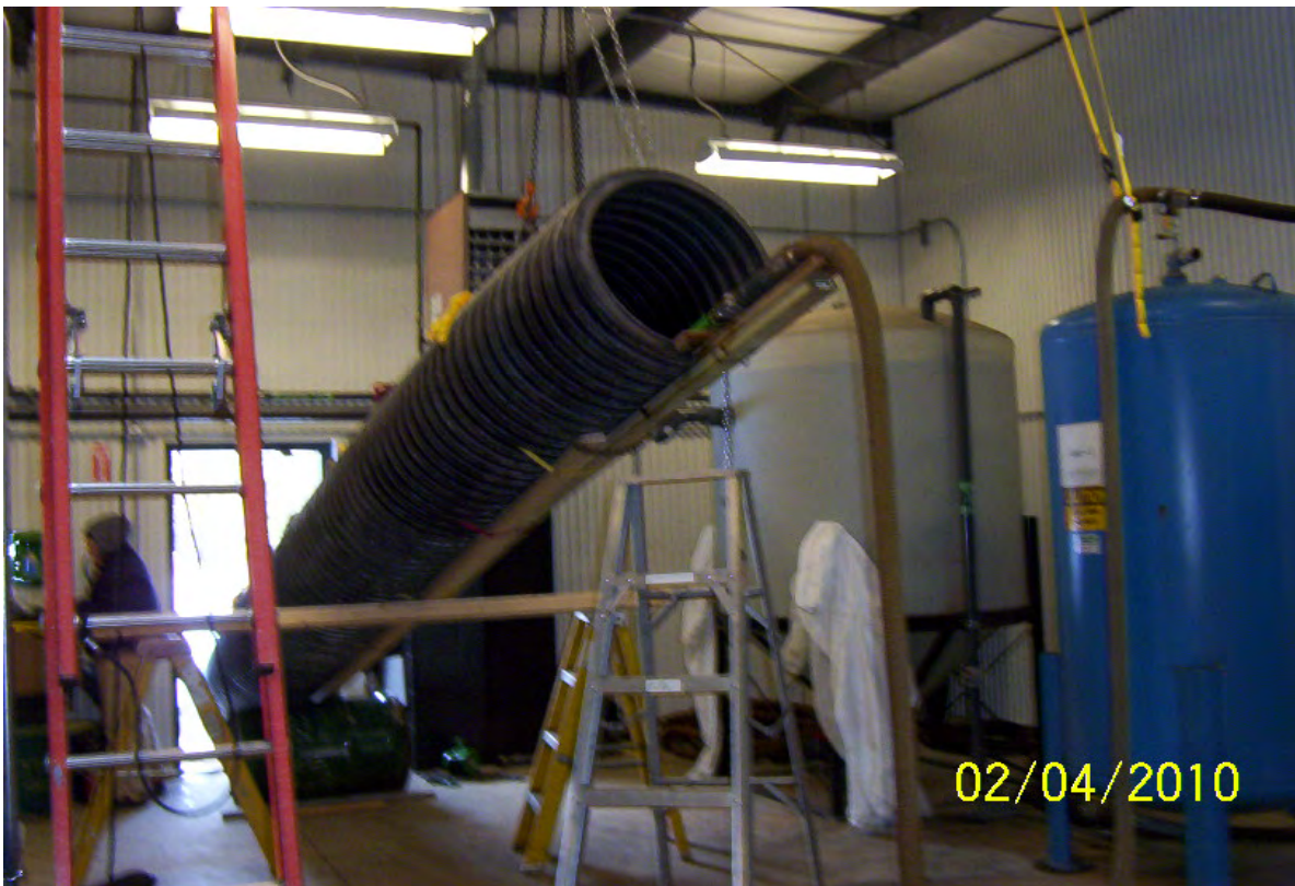
Photo 2: Pipe Slope 3 to 1
