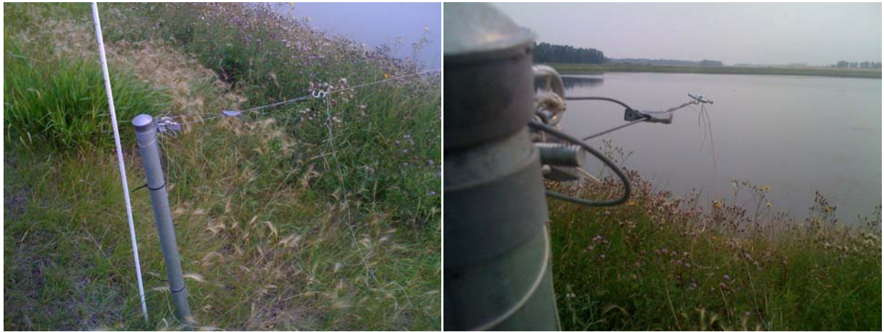
Figure 4: Bird Prevention Wires (EIA, Alberta, Canada)
