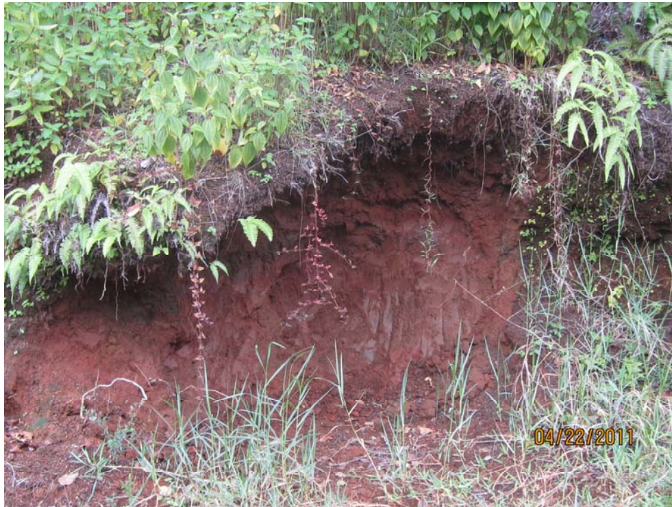
Plate 7. Sample S-3 was taken from this road cut. At the time when the soil was sampled the exposed slope was standing vertical.
