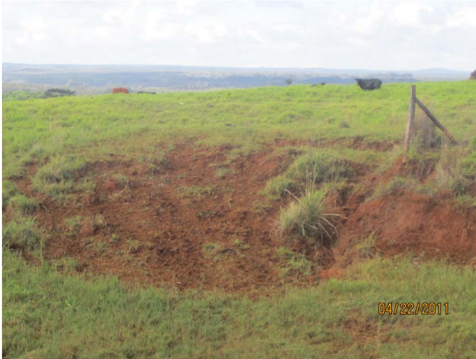
Plate 2. Photograph of Minor Slide Developing in Pahala Ash.
