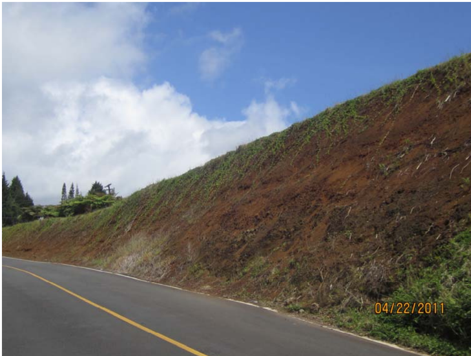
Plate 3. Photograph of a Steep Road Cut Through Weathered Bedrock and Pahala Ash on Kaiwiki Road.
