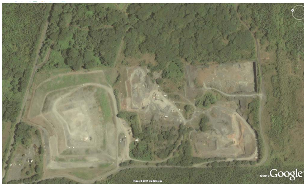
Figure 2: Aerial Photo of South Hilo Landfill
